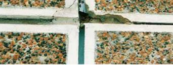
The solution with EGOSIL TAPE elastomer joint tape
