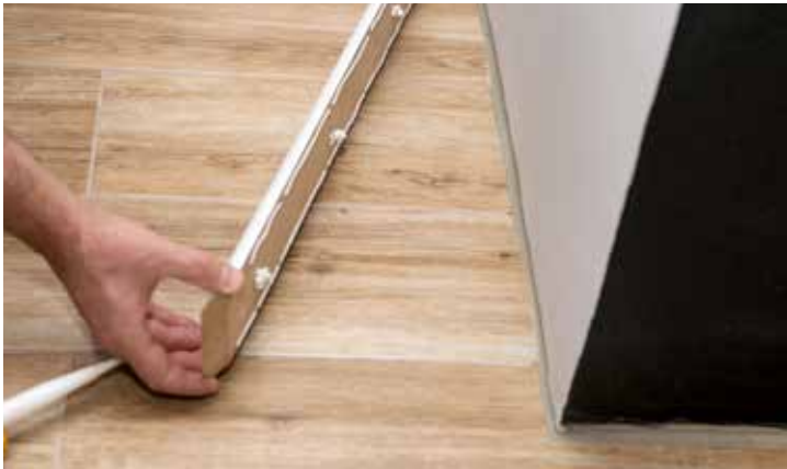
Adhesion of skirting boards in dry-wall and masonry construction with EGO SMP 805
