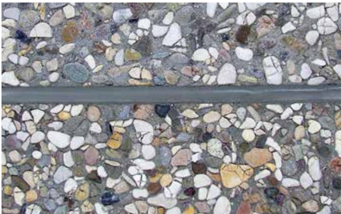
Floor joints that can be walked on in an exposed aggregated concrete surface EGO SMP 805
