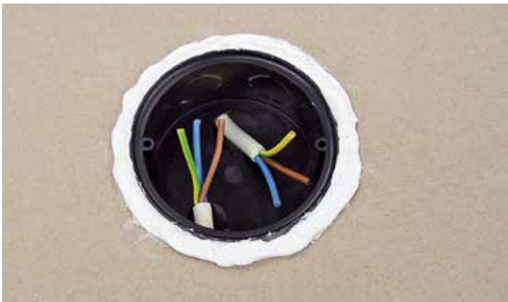
Attachment of electrical sockets with EGO SMP 805 in wall recesses
