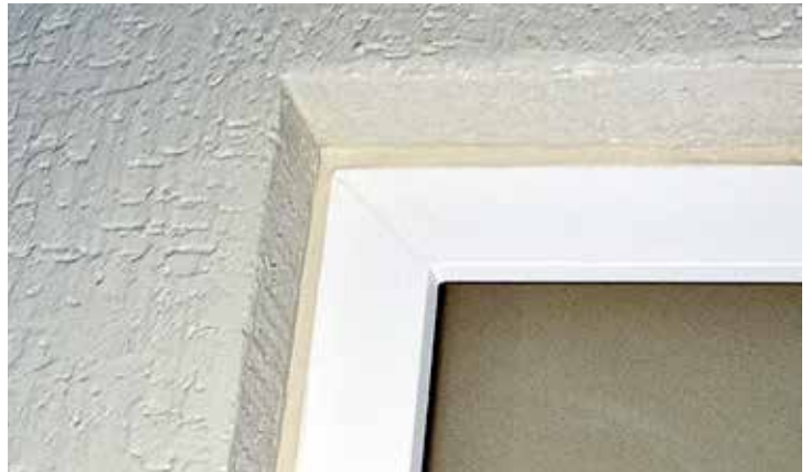
Exterior window connection joints with EGO SMP 818
